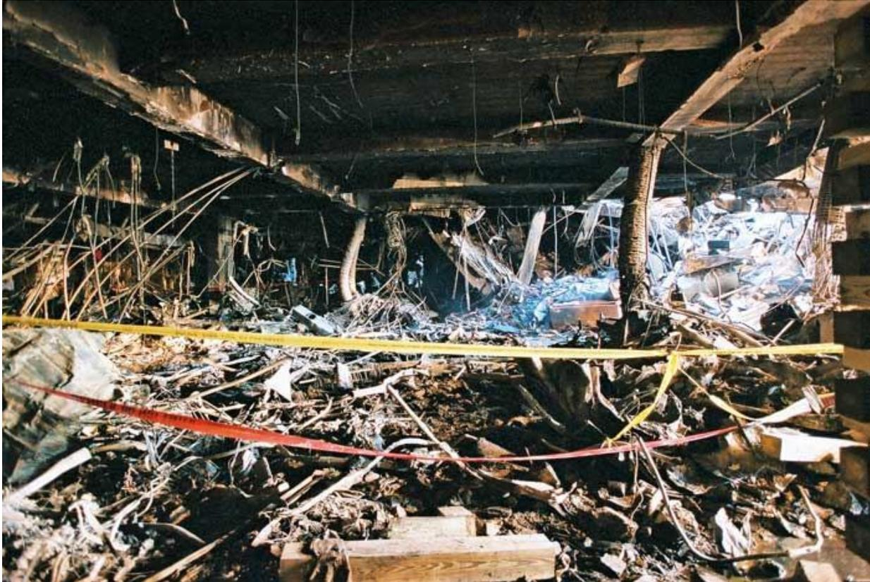
In this photo we see a massive amount of debris at the ground floor level. The plane would have passed from right to left across this scene and we observe that the support columns all appear to have been pushed to the left, as would be expected. In one case only the reinforcing rods are still visible.
