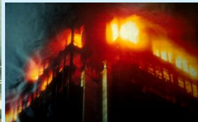
First Interstate Bank fire, close-up
