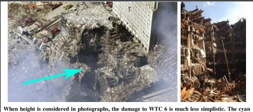
When height is considered in photographs, the damage to WTC 6 is much less simplistic. The cyan arrow marks the same location in the left photograph as well as the previous aerial photograph.
