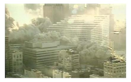
5. WTC 7 was 174m high and had 47 storeys. Study of photographs and diagrams in the FEMA report shows that there was additional height in floors near the ground, in the middle and at the top. This additional height was equivalent to about 1.7 storeys, thus the height of a standard storey was 3.67m.
