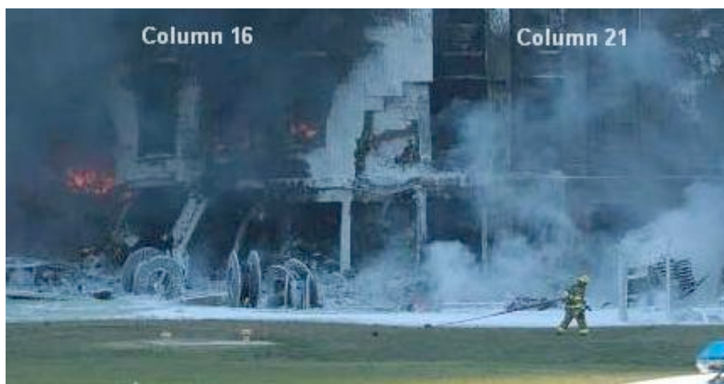
Figure 4. Impact region with cable spools.
