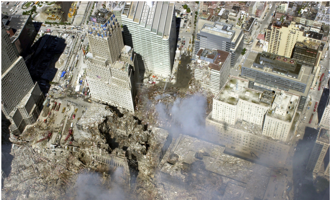
WTC6 (at lower left) and WTC5 (at lower right) after the collapse of both towers
