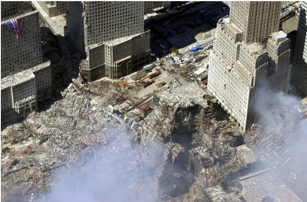
WTC6 after the collapse of the Twin Towers exhibiting heavy damage to three sides of the building deepening in the center
